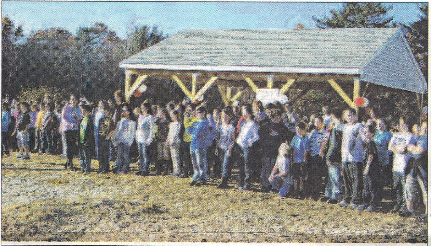
Students gather around the newly built shade structure at Hopkins Hill Elementary. The structure which will keep kids safe from the sun's UV rays was built under the concerted efforts of parents, businesses and students.
